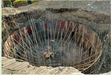
Construction of the Water Harvesting Tank
